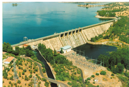
Photo 4: Orellana – a reservoir project in Spain
