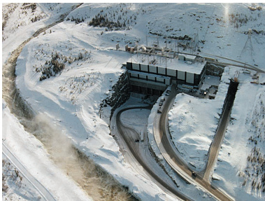
Photo 5: Brisay – a single purpose project in Québec, Canada
